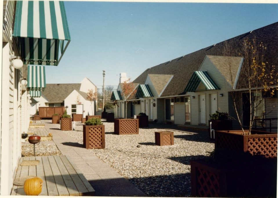
Central patio of residential area. Note use of gravel and wooden porches at each apartment entry to protect roofing membrane.
