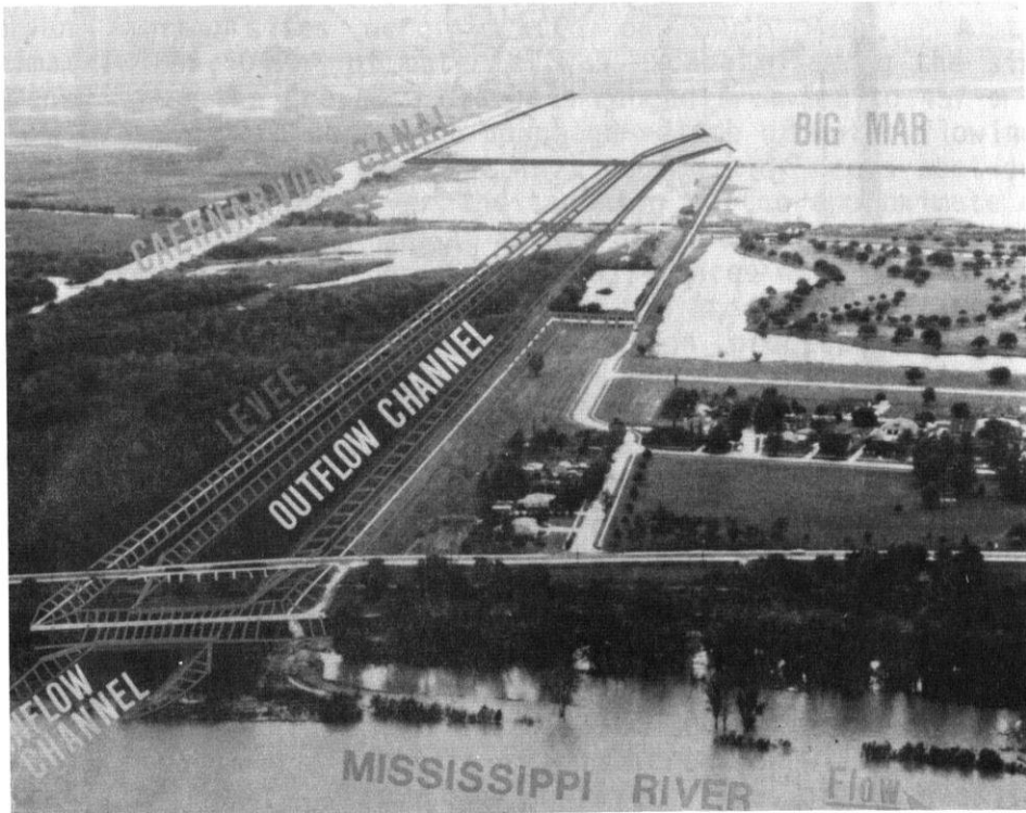
Figure 2. Conceptual view of the proposed Caernarvon freshwater diversion structure (reprinted from U.S. Army Corps of Engineers News Release, June 17, 1987).
