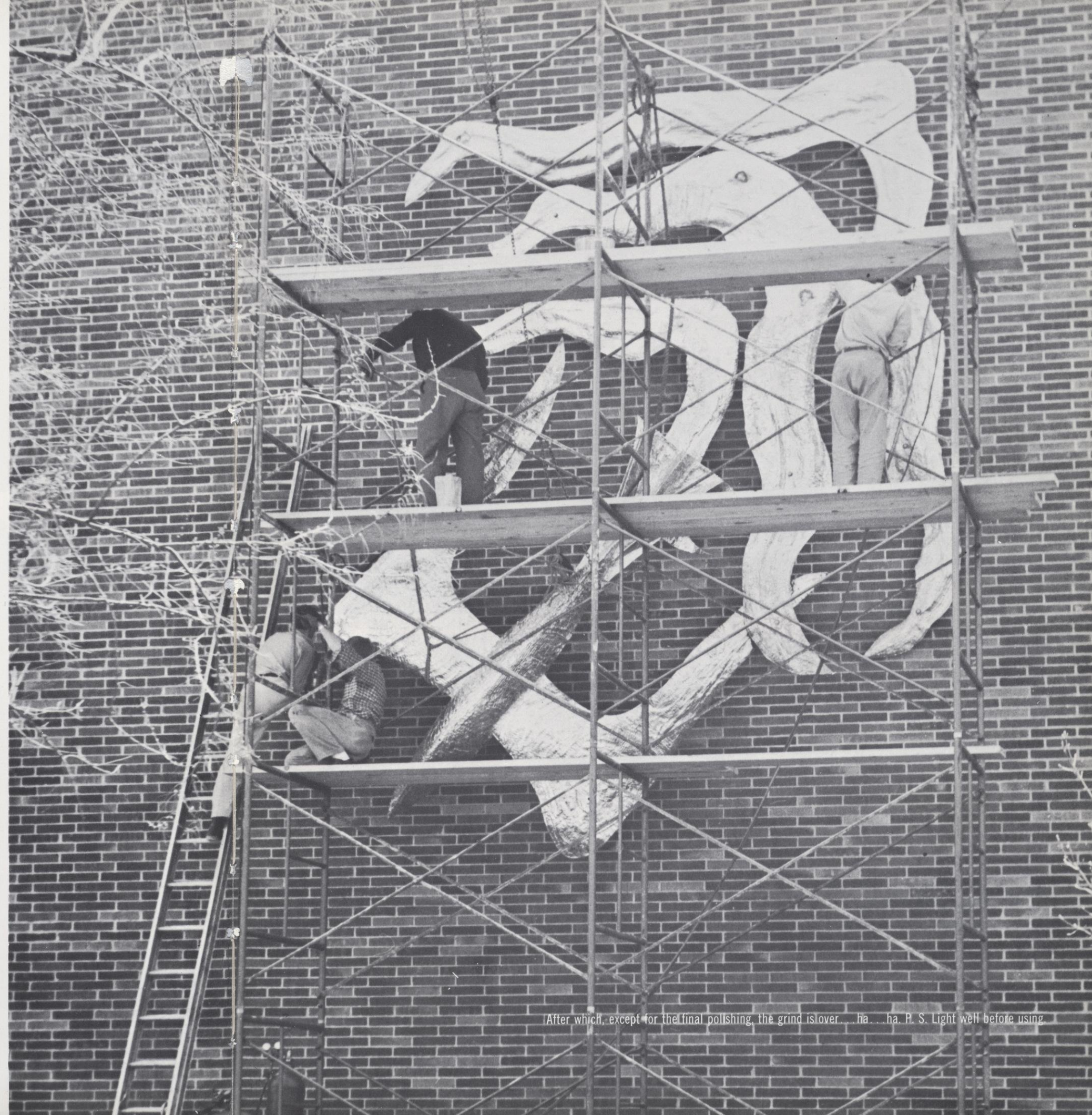
Finally, bolt and weld it to the wall.
