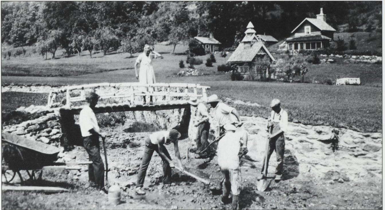
Mother Anne Dable supervising stream bed construction, c. 1933. Little Norway Collection.
