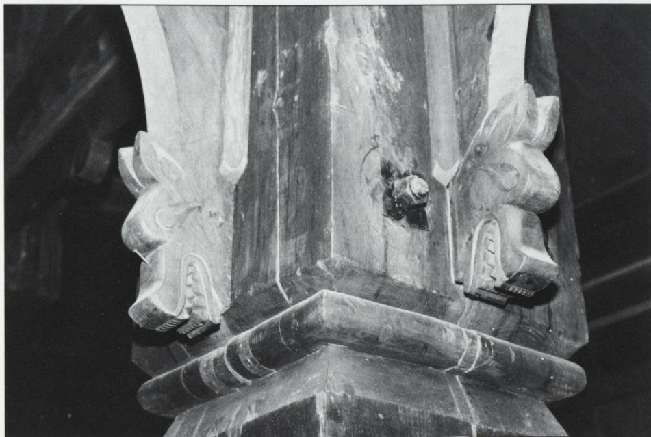
Dragon heads form the ends of the quadrant brackets. This detail is a direct influence of architect Hansteen's involvement with the Gol Stave Church restoration project.
