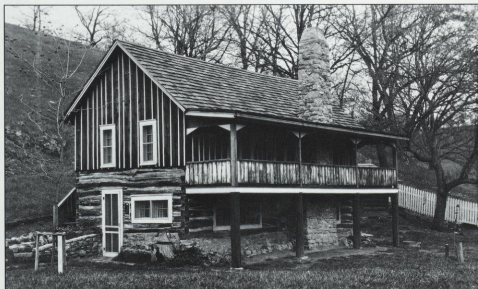
Completed cattle and sheep barn with porch and stone chimney added.
