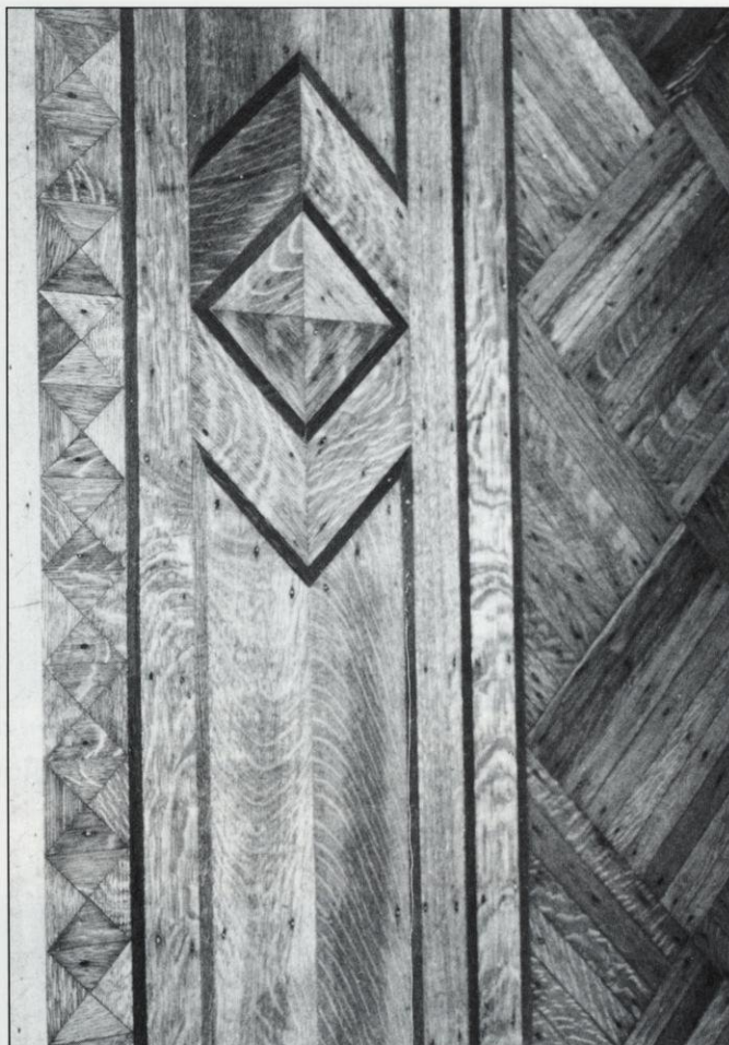
Detail of parquet floor, contemporary to the 1890's.
