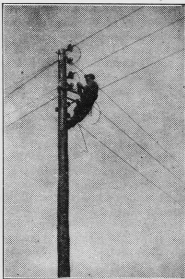
Two phase double dead end construction.—Rock project.
