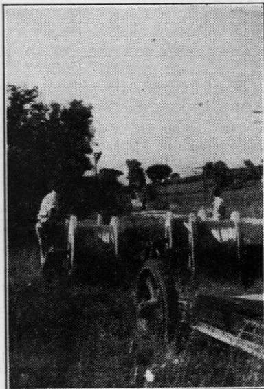
Stringing conductor. Rock project.
