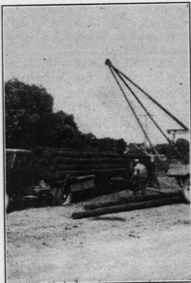
Pole distribution and setting. Rock project.
