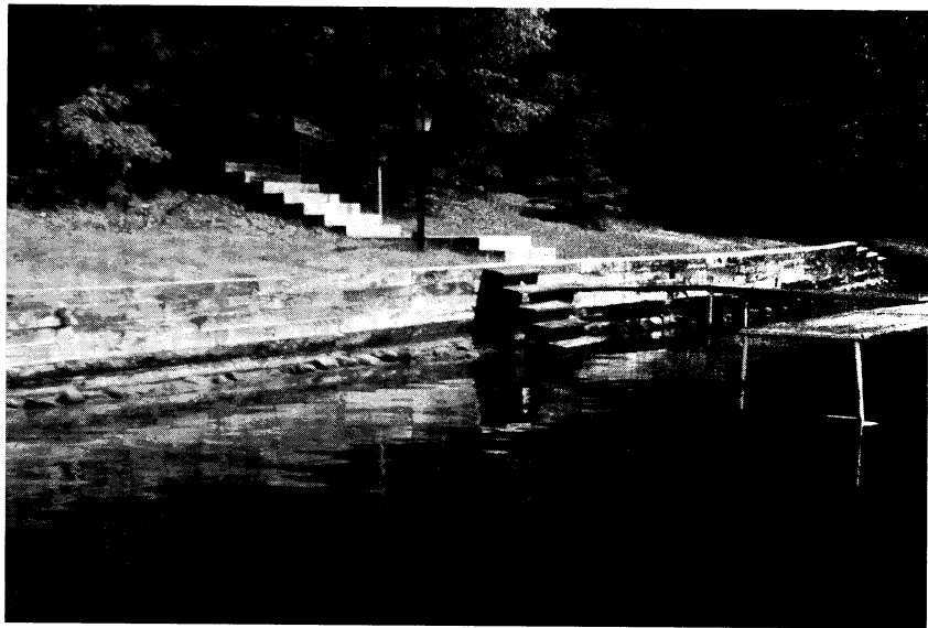
A wooden seawall built of horizontal railroad ties beside a sectional pier on Upper Gresham Lake, Vilas County, Wisconsin.
