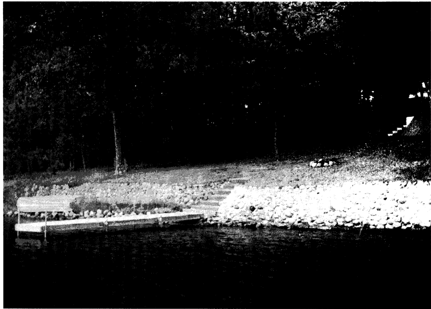
A seawall of mortared stone protecting a lakeside lawn on Bass Lake, Oconto County, Wisconsin.
