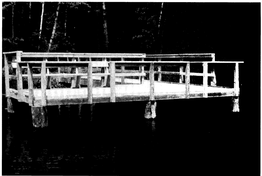
A permanent pier built of chemically treated lumber and accessible to all anglers on Upper Gresham Lake, Vilas County, Wisconsin.
