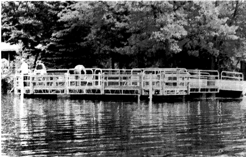
A seasonal pier built of aluminum railings and sectional decking accessible to all anglers on Half Moon Lake, Eau Claire County, Wisconsin.
