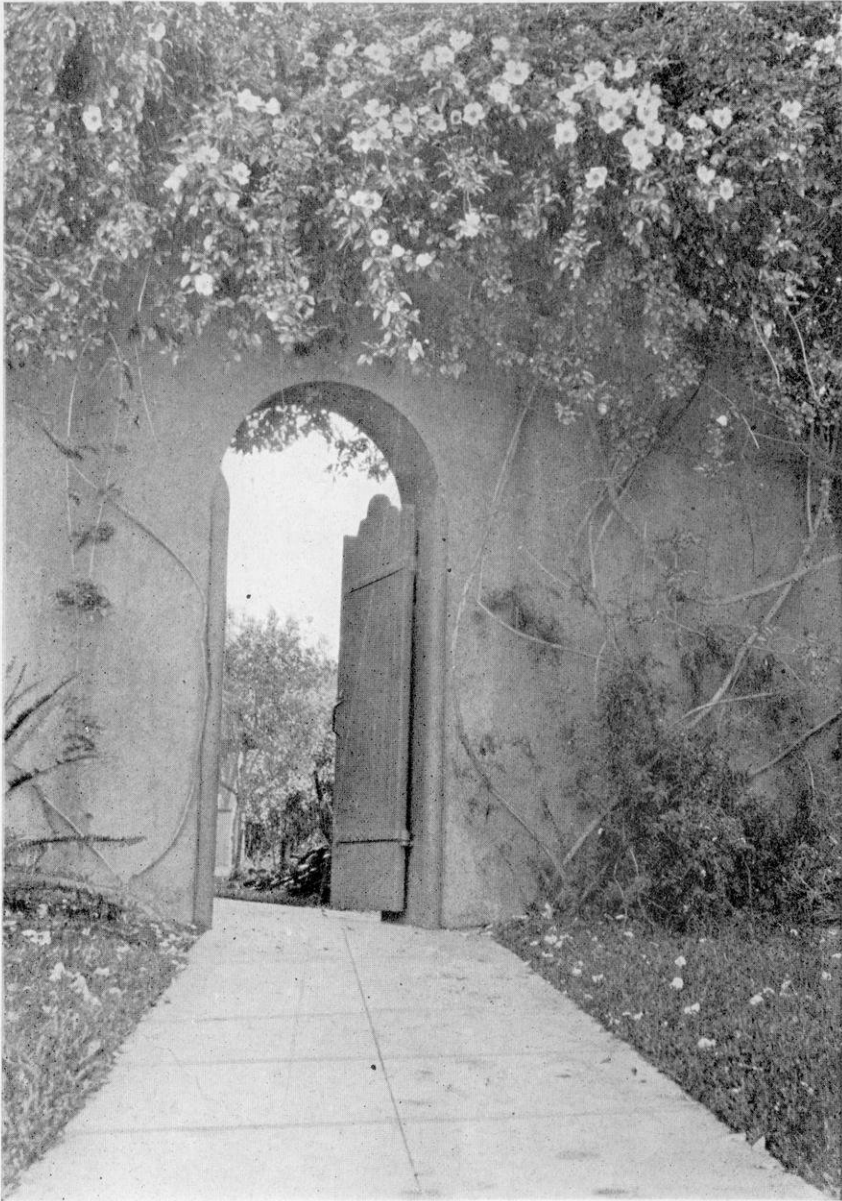
"THIS CEMENT WALL WAS BUILT AFTER THE FASHION OF THE OLD MISSION WALLS: THE GATE IS WOOD BOUND WITH IRON BANDS, AND THERE IS A SPACE OF BLUE BETWEEN DOOR AND CEMENT ARCH."
