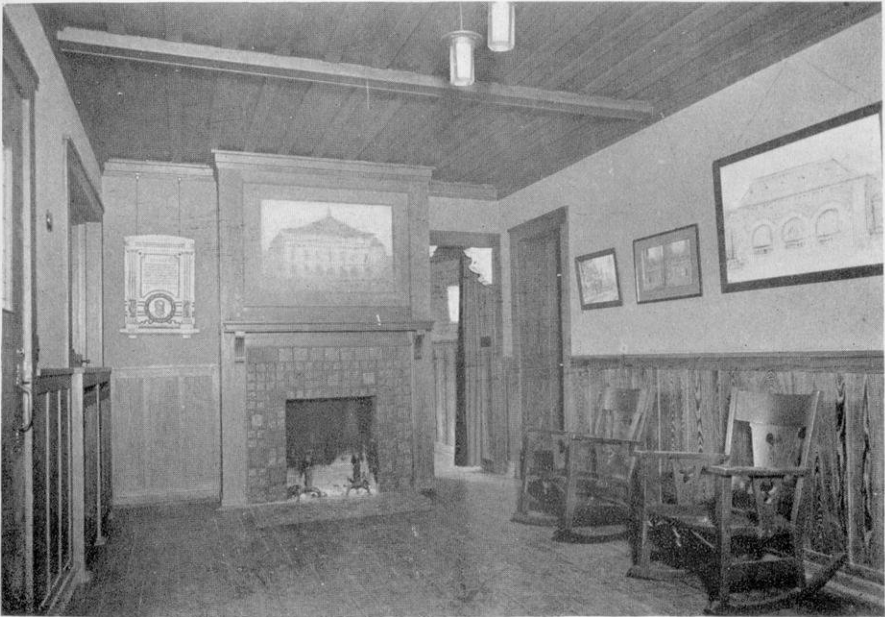
PRIVATE OFFICE, SHOWING FOUR-FOOT WAINSCOT OF CYPRESS, TREATED IN JAPANESE MANNER. OUTER ROOM, CONNECTING WITH PRIVATE OFFICE.
