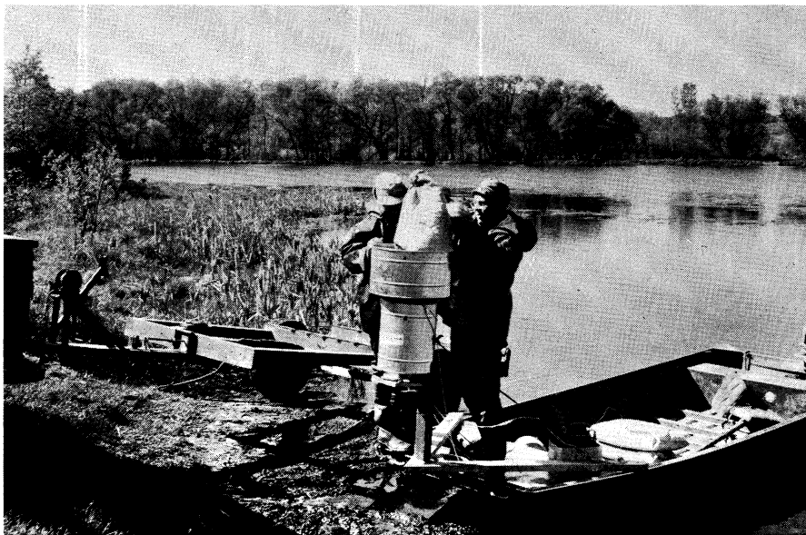
Granular applying equipment. This relatively inexpensive equipment is used only on large projects. Areas of 10 acres or less are most usually treated by simple hand-broadcasting techniques.
