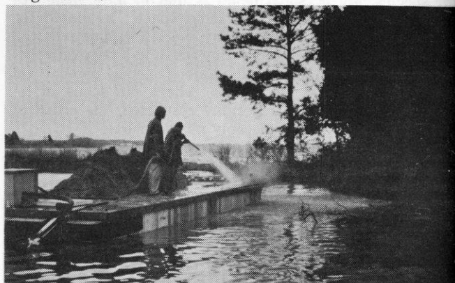
Figure 1. Building graded tidal flat by barging in new substrate.
