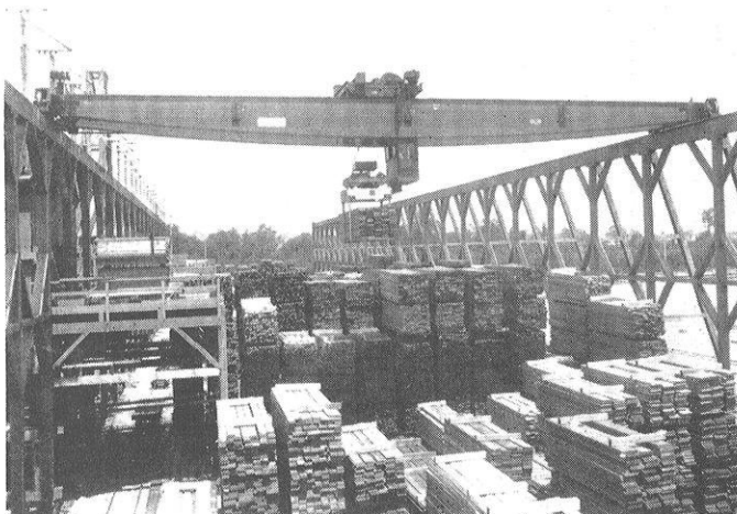
Fig. 4. Lumber-handling crane showing lumber grapple, bridge and trolley collectors.
