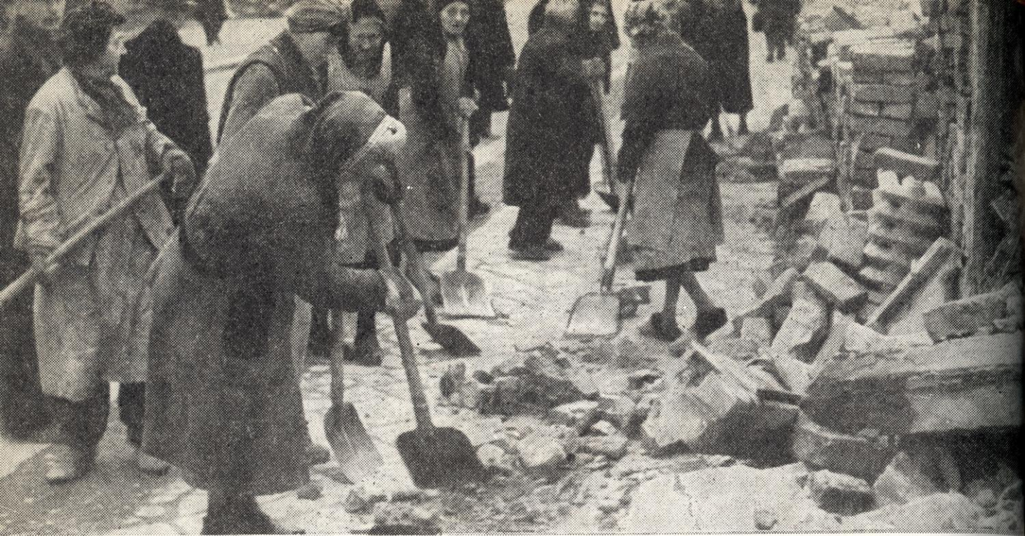
Berlin women, using shovels, take the place of scarce machinery in clearing debris in front of bombed-out buildings. (DENA-Bild)
