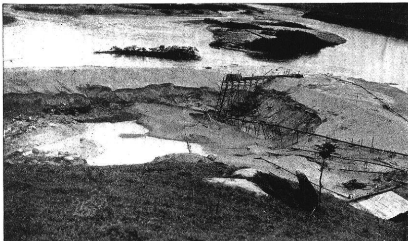
FIG. 2: In the Porce River, work is conducted to exploit the ancient river bed; then the river is run through the holes made, and the actual bed is worked.
