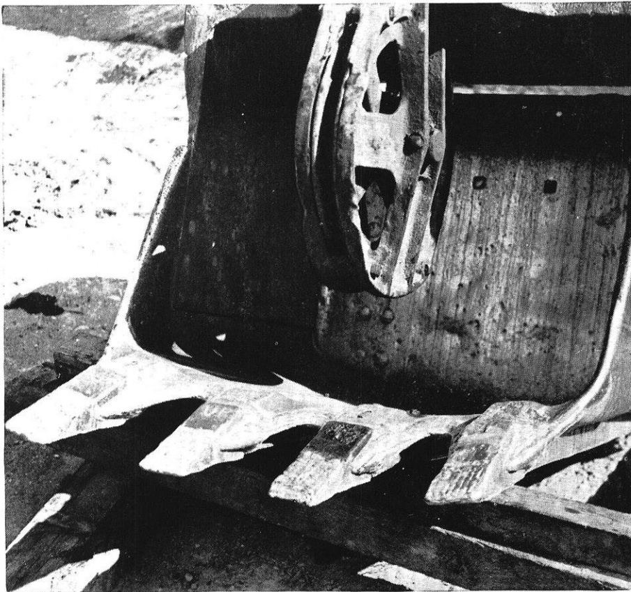
INTO THIS YAWNING CAVITY goes the dirt to make Grand Coulee Dam. Bucket front and teeth were hard-faced by welding. The result of this wearproofing was six months' service on Bonneville Dam, and many more months of trouble-free, repairless service on Grand Coulee.
