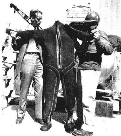
Fig. 1. This special "wet" suit circulates warm water over the diver's body to keep him warm in the cold depths.
