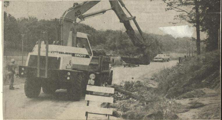
County workers work to keep Hwy. 191 between Dodgeville and Hollandale open after heavy rains caused mud to flow onto the road at various locations. The footings were washed out on a box culvert just north of the 191-CTH "W" intersection last Friday, causing 191 to be closed to traffic over the weekend.
