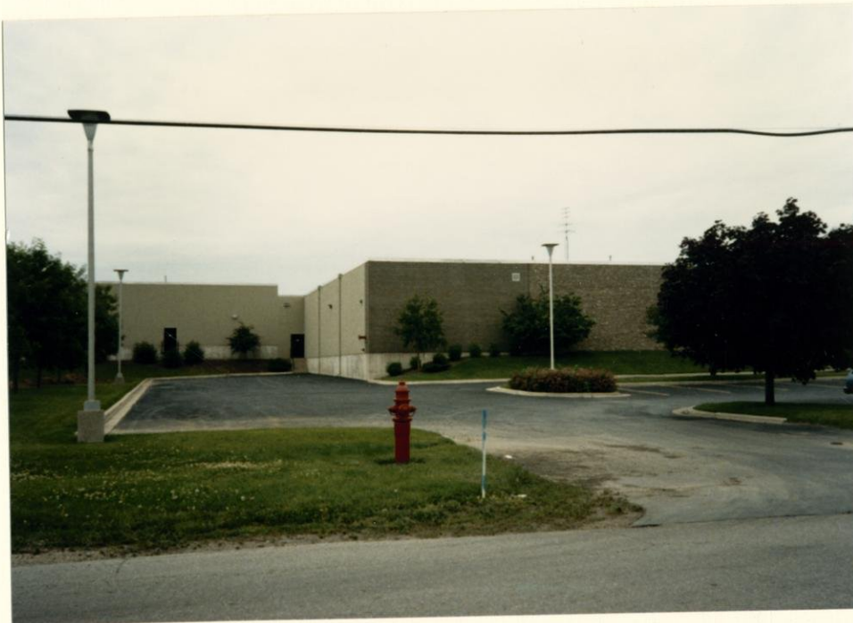
View of southeastern access to Phillips from Raywood Road. This is the only access which will remain after the taking.
