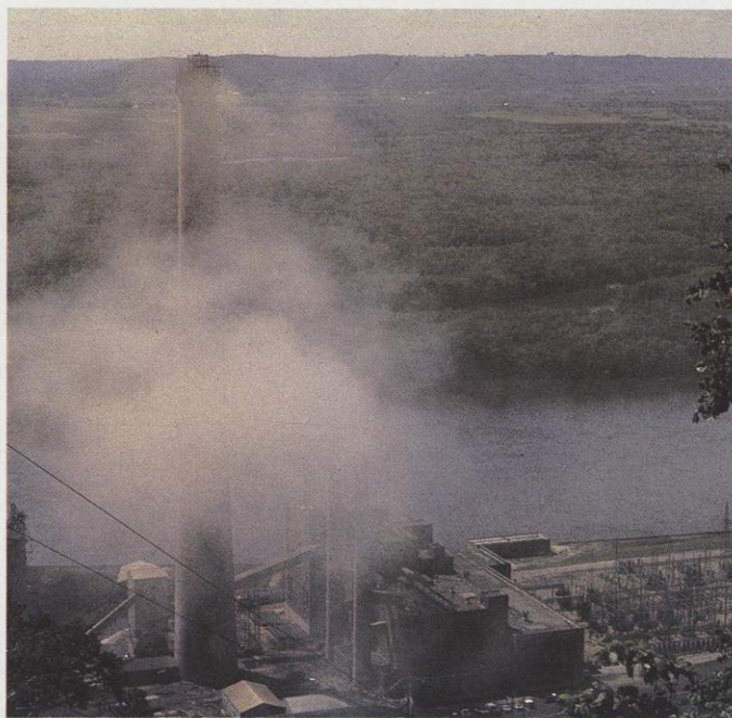
Sulfurous smoke “downwashing” from an Alma power plant in 1973 carried pollutants to the ground. Switching to lower-sulfur coal, installing precipitators to trap sulfur and raising stacks reduced pollution near the plant.
