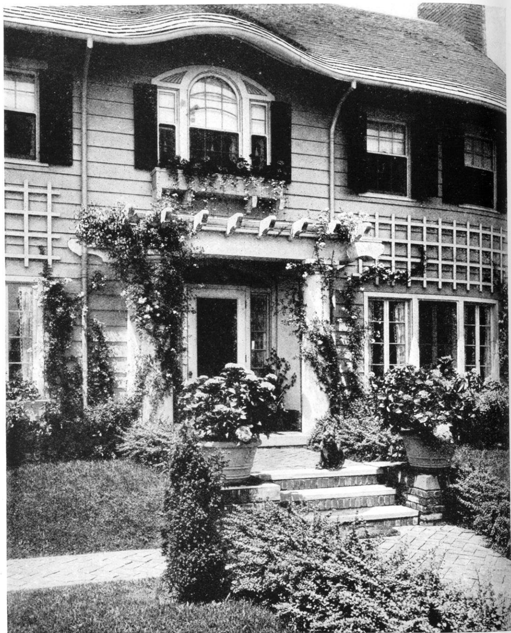
LATTICE IN THE FORM OF LADDERS and incorporated directly in the house construction as has been done in this house, designed by Frank D. Meade and James R. Hamilton for "Gray Gables," the home of J. H. Woods, Esq., Clifton Park, Lakewood, Ohio, makes an extremely decorative effect.
