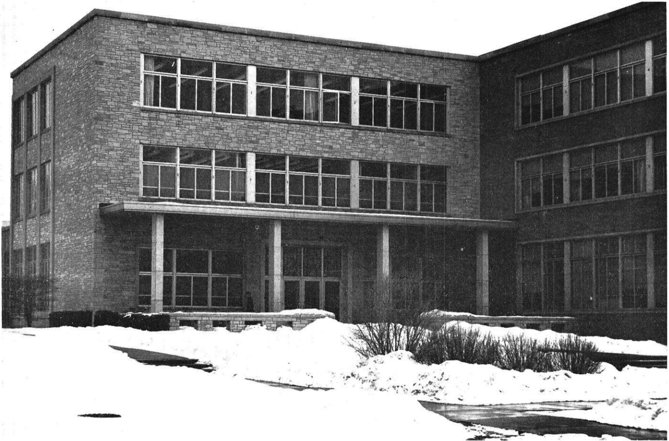
The Electrical Engineering Building.
