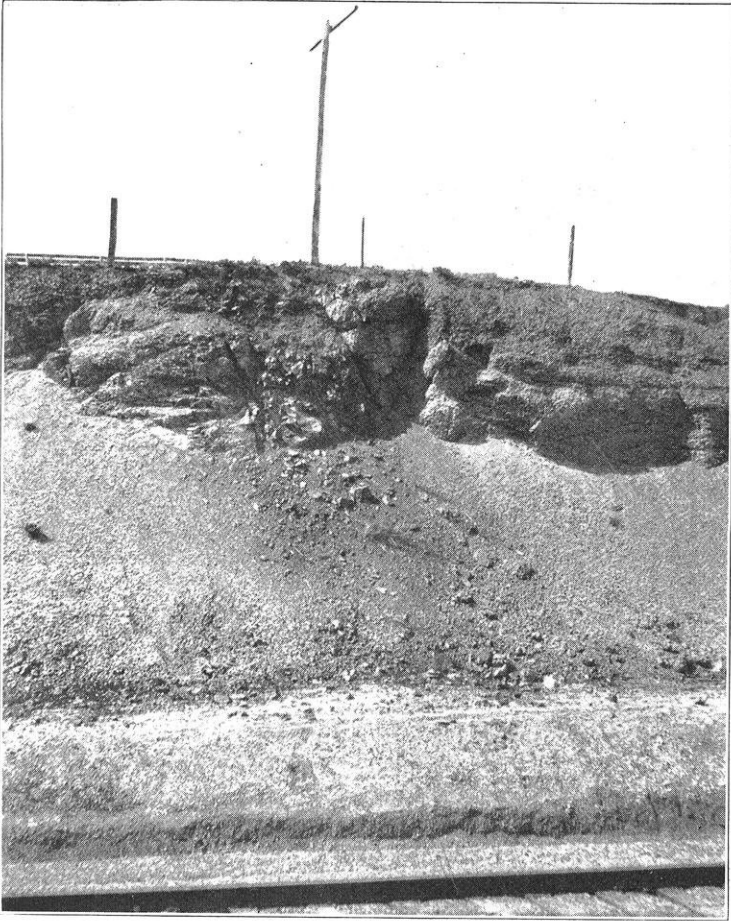
Fig. 3. Side of a railroad cut in the deeply rotted granite near Sherman, Wyoming. Shows a basalt dike cutting the original granite with slopes of loose gravel from both.)
