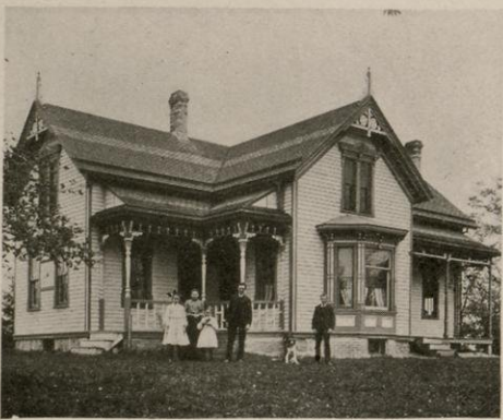
RESIDENCE OF AUGUST HALTER Caledonia Township
