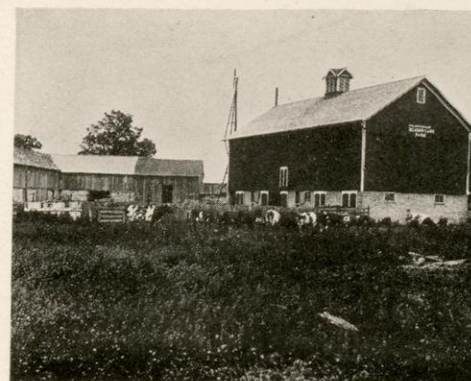
BARN OF D. M. CUNNINGHAM Rochester Township
