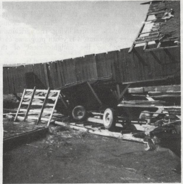
Kenneth Gumz farm - Tornado damage Sept. 28, 1971
