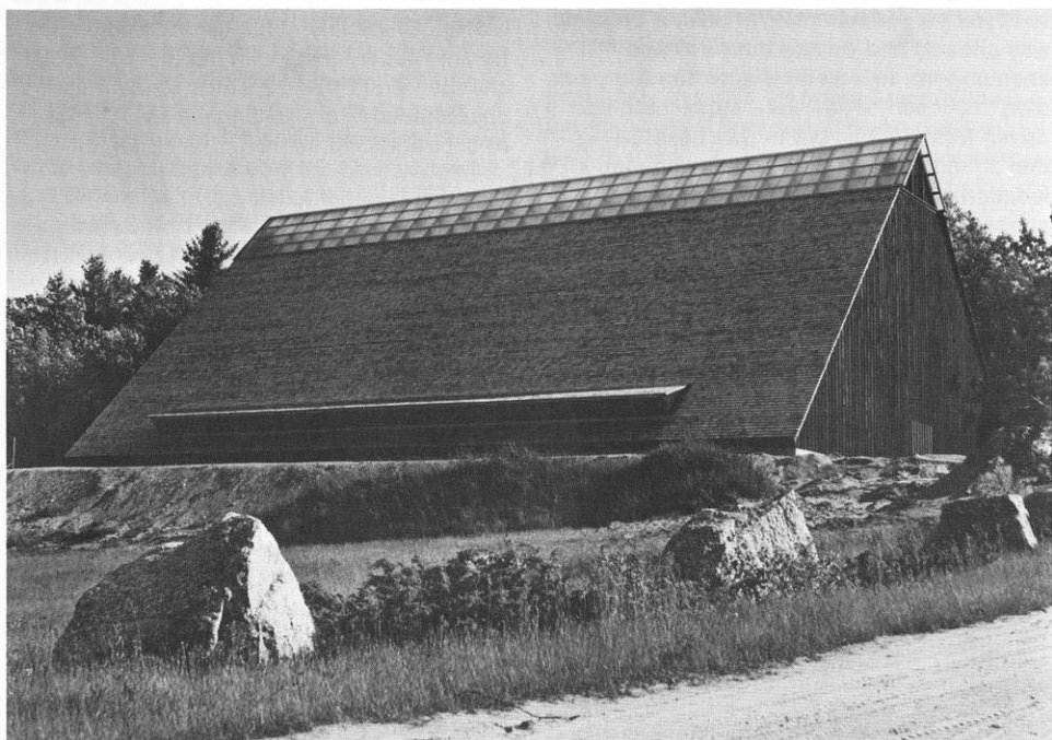
Field House, Camp Kenwood, Potter Place, N.H. Architects: Goody & Clancy; Joan Goody, Partner-in-charge. This simple structure covers a large (70' x 110') area with an extremely economical structural system. It houses rainy day and evening athletics for a large camp.
