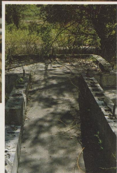
Abandoned miniature golf course will be removed and wetlands restored.
