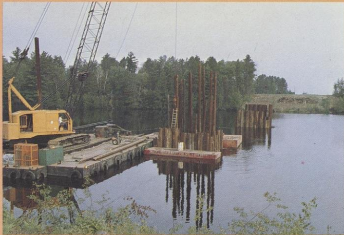
Early bridge construction techniques often caused more damage than necessary to natural resources because engineers first build an island on the streambed from which to operate machinery. This is now avoided whenever possible. The environmentally acceptable technique shown here was used by DOT on the new highway 51 bridge over the Wisconsin River at Tomahawk where machinery is operated from a raft. DNR and DOT also worked together here to minimize boating hazards during construction. Photo by Dale Lang
