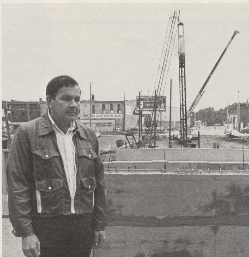
The author at a bridge construction site on Farwell Street in Eau Claire.
