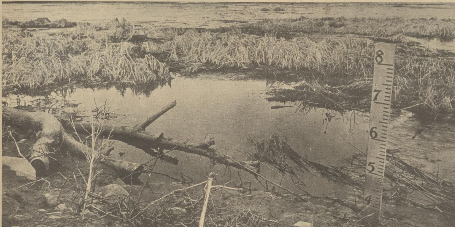
LEFT: PARTIALLY treated sewage flooded into the Nine Springs creek and the Yahara river Sunday after the earth dike surrounding Madison's sewage settling pond gave way after a heavy rain. The level of the mile square pond was down almost two feet while the escaping sewage resulted in a heavy fish kill and strong stench along the length of the rivers.
