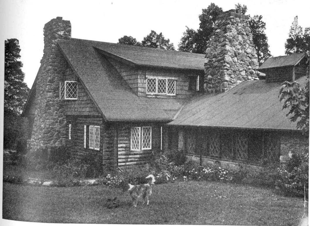
A VERY PLEASING USE OF IRREGULAR FIELD STONE WITH STUCCO ABOVE IS SHOWN IN THIS HOUSE AT MERION, PA., DESIGNED BY DAVID KNICKERBACKER BOYD.
