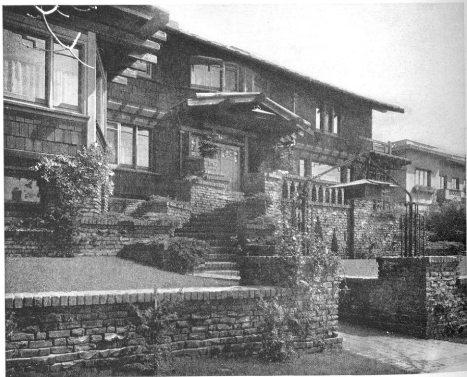
ANOTHER VIEW OF MR. NEILL'S HOME, THE GARDEN WALL OF WHICH IS SHOWN ON PAGE 534: AN INTERESTING EXAMPLE OF BRICK AND COBBLESTONE. A HOUSE IN BERKELEY, CALIFORNIA, DESIGNED BY GREENE AND GREENE: NOTE THE IRREGULAR PLACING OF THE BRICKS, AND THE TERRACED ENTRANCE.
