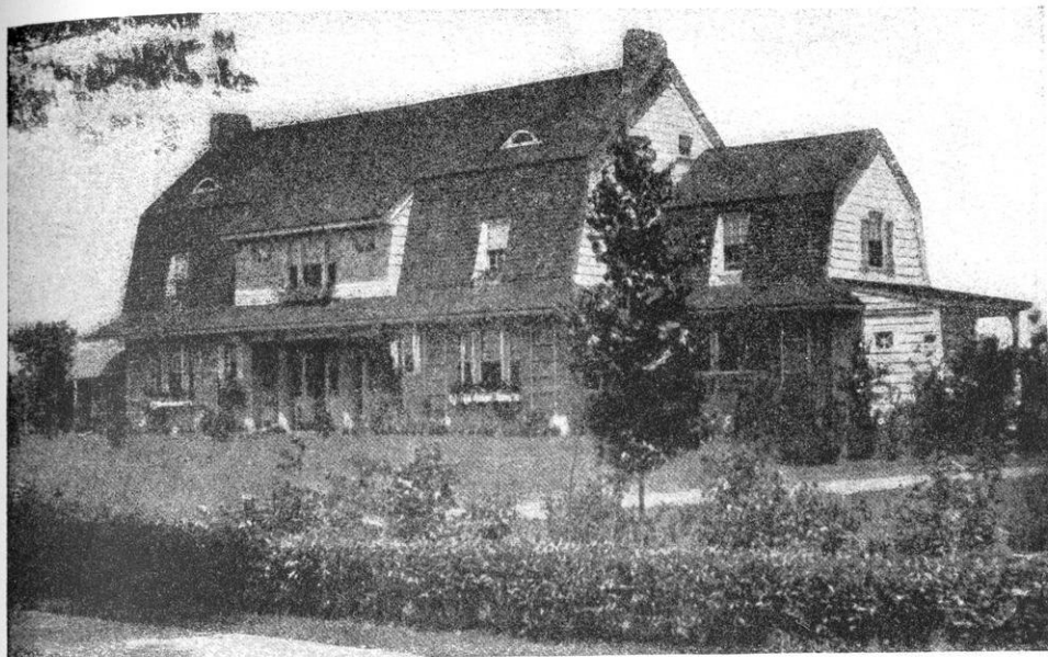
THE WIDE CLAPBOARD WALLS AND SHINGLED GAMBREL ROOFS OF THIS DIGNIFIED, HOSPITABLE-LOOKING HOUSE ARE WELL SUITED TO THE DESIGN: IT IS THE HOME OF HENRY S. ORR AT GARDEN CITY, LONG ISLAND, AND IS AN EXCELLENT INSTANCE OF THE WORK OF AYMAR EMBURY II, WHO HOLDS TO THE BEST COLONIAL AND DUTCH TRADITIONS.
