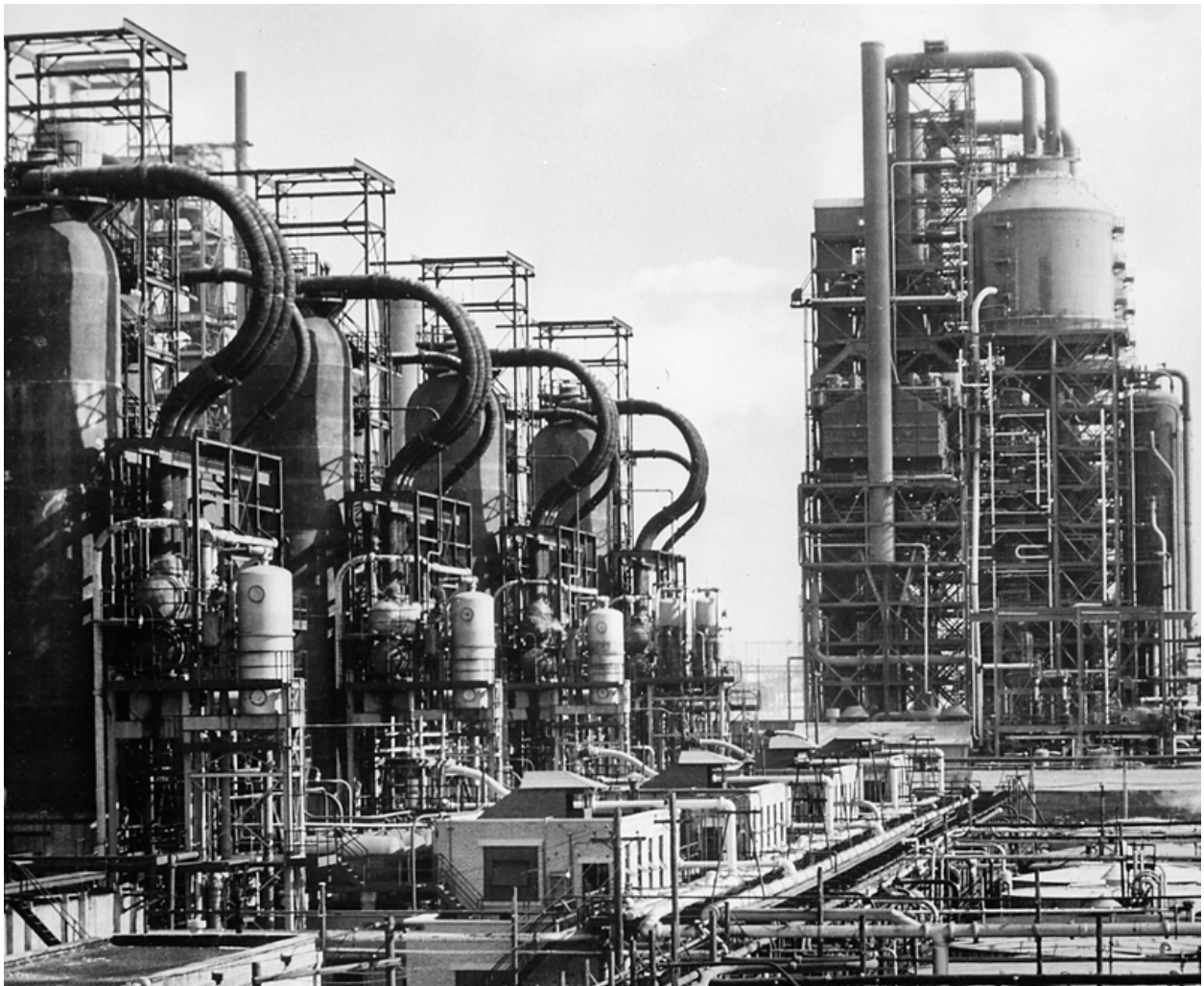
Figure 4-1: Open architecture on display at the Baton Rouge Esso oil refinery c. 1945. Note the capsule-like reactor vessels of the cracking units at left. Photo courtesy of the National Archives and Records Administration, catalogued under identifier 535733.
