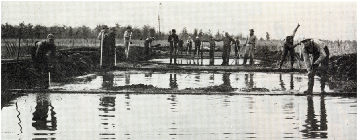
Figure 3-4: Building a new board road after the previous one had collapsed in the marsh, c. 1942. Image from: Gordon B. Nicholson, "Road Construction in Swamps Presents Difficulties." Photo used with permission.
