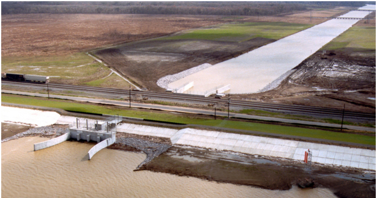
Figure 5-2: Davis Pond freshwater diversion sometime after completion in 2002. This structure was built to defend against saltwater intrusion by diverting freshwater from the Mississippi into the coastal marshes. Though similar in principle, sediment diversions are constructed differently in order to maximize the amount of suspended sediment in diverted waters. The Davis Pond structure (just downriver from the site of 1884 Davis Crevasse discussed in chapter one) has a maximum capacity of 11,000 cubic feet of water per second (cfs), an order of magnitude smaller than some of the 250,000 cfs sediment diversions proposed in the 2012 Coastal Master Plan. Photo courtesy of the US Army Corps of Engineers.
