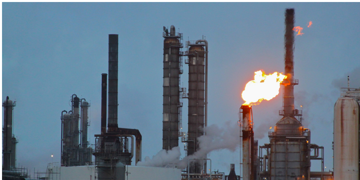
Figure 4-2: A Shell refinery in Deer Park, Texas, March 16, 2012. The tallest stack with a flared base on the right is a feed heater. The two center stacks are fractional distillation columns. The white vertical capsule at the far right of the image is likely a reactor vessel of some sort. Also note the flare stack. Photo by Roy Luck, Creative Commons Attribution 2.0 Generic License .
