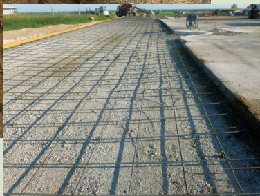
Addition to an existing feed pad, which will divert leachate to a reception tank.
