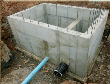
Feedpad leachate reception tank to manure storage.
