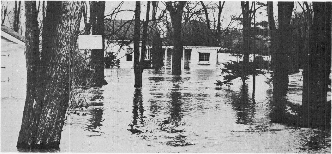
Figure 8 BASEMENT FLOOD DAMAGE
