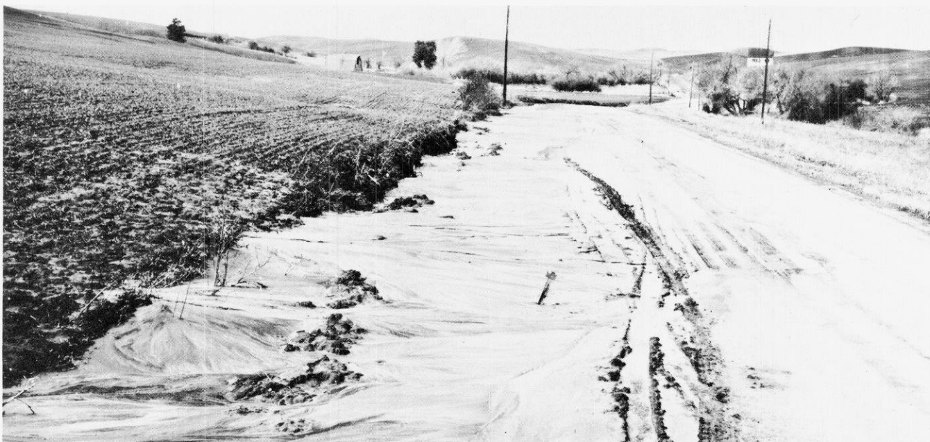
Figure 17 SILTING OF DRAINAGE DITCHES
