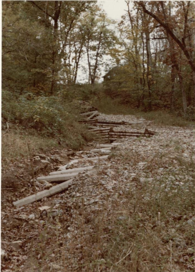
Storm Water Management Area for Park View Heights Subdivision
