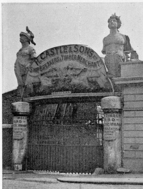
Messrs. Castle and Sons, Baltic Wharf, London, Main entrance
