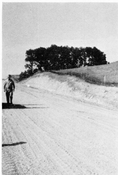
Figure 15. Road cut through loess-covered till showing thickening of leached loess covering down-hill (toward the foreground). The toposequence is from Theresa silt loam on the ridge to Dodge silt loam in the foreground.
