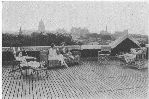
ON THE ROOFTOP
