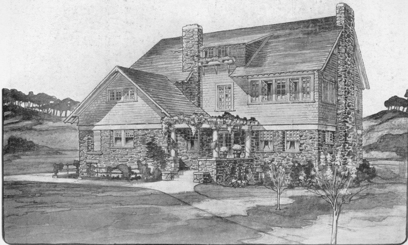
REAR ELEVATION OF CRAFTSMAN HOUSE SHOW- ING INTERESTING ROOF AND PERGOLA-PORCH.
