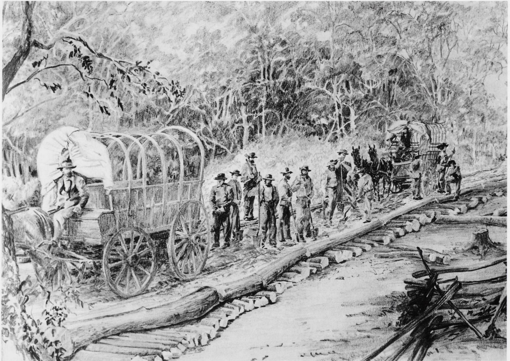
A practical but time-consuming way to make marshes passable was to construct corduroy roads out of trees felled in local forests.
