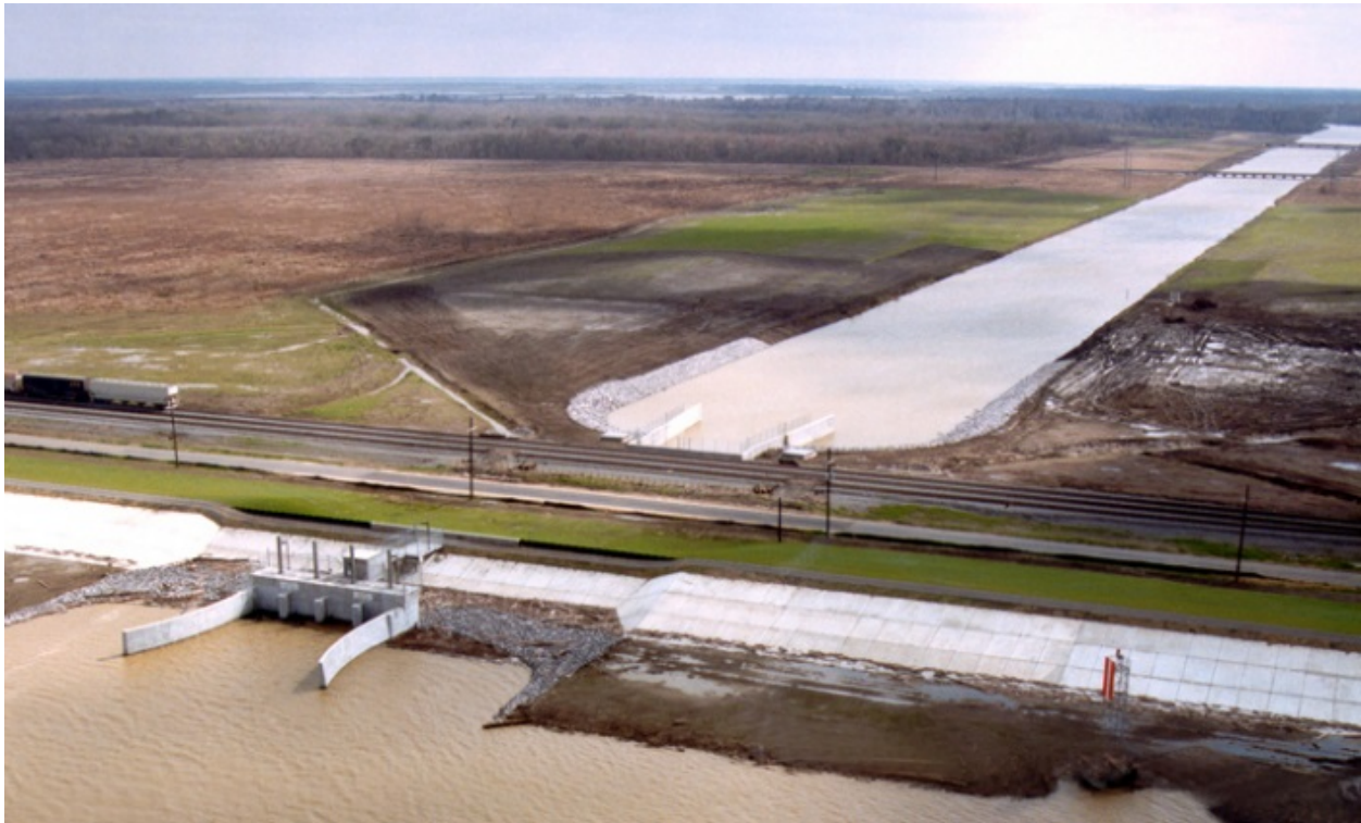
Figure 4. The Davis Pond freshwater diversion. Sediment diversions will look similar, but are designed specifically to move as much sediment as possible into degrading sub-basins. Source: Corps of Engineers.
