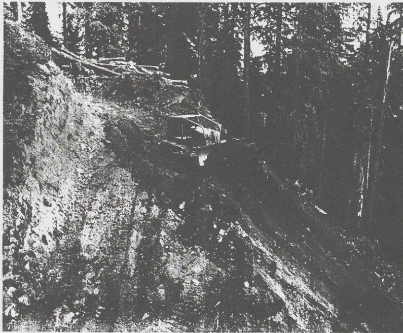
Caterpillar tractor building a road on the Mt. Baker-Snoqualmie National Forest. Photo taken by Donald Stickney in 1957. Photo credit: USDA Forest Service
