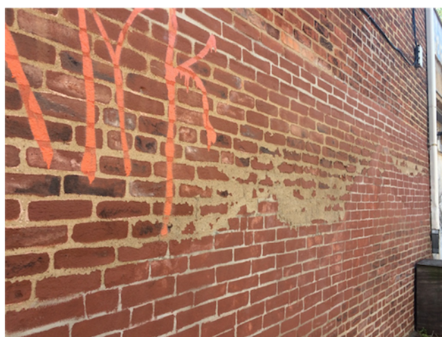
Figure 17. A concrete wall painted to look like historic red brick in Naylor Court. Photo by author, 2017.
