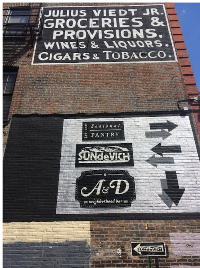
Figure 16. Signage for new and old businesses mix on the facades of Naylor Court buildings. Photo by author 2017.
