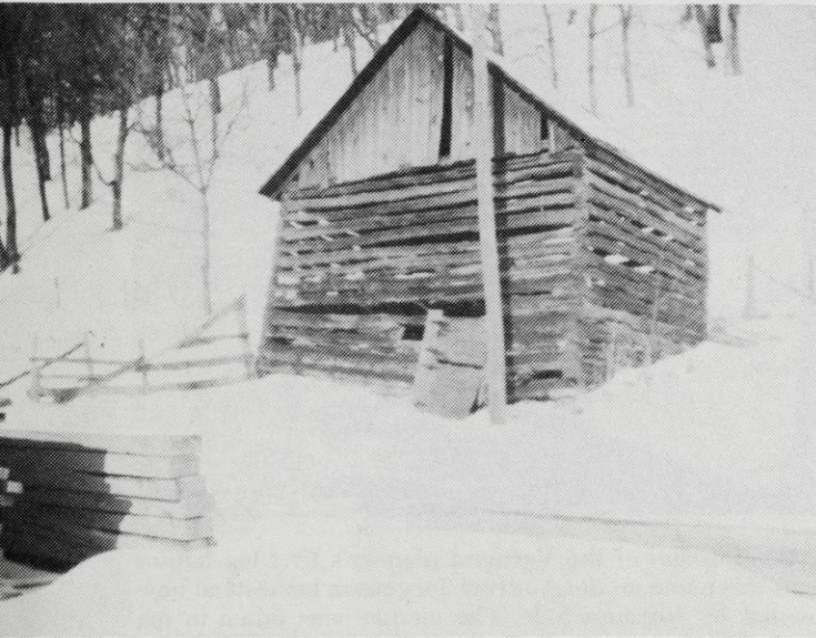
The chinking between the logs is all but gone on the Jorgenson barn by 1940.
