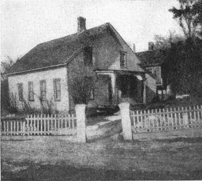
THE OLD FARMHOUSE AS IT LOOKED BEFORE MR. HUTAFF TOOK IT IN HAND—A SOMEWHAT DRAGGLED AND GLOOMY STRUCTURE.
