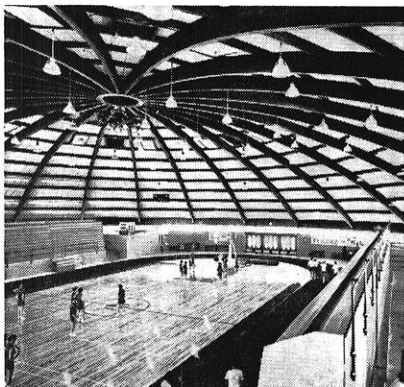
Laminated wood arches
