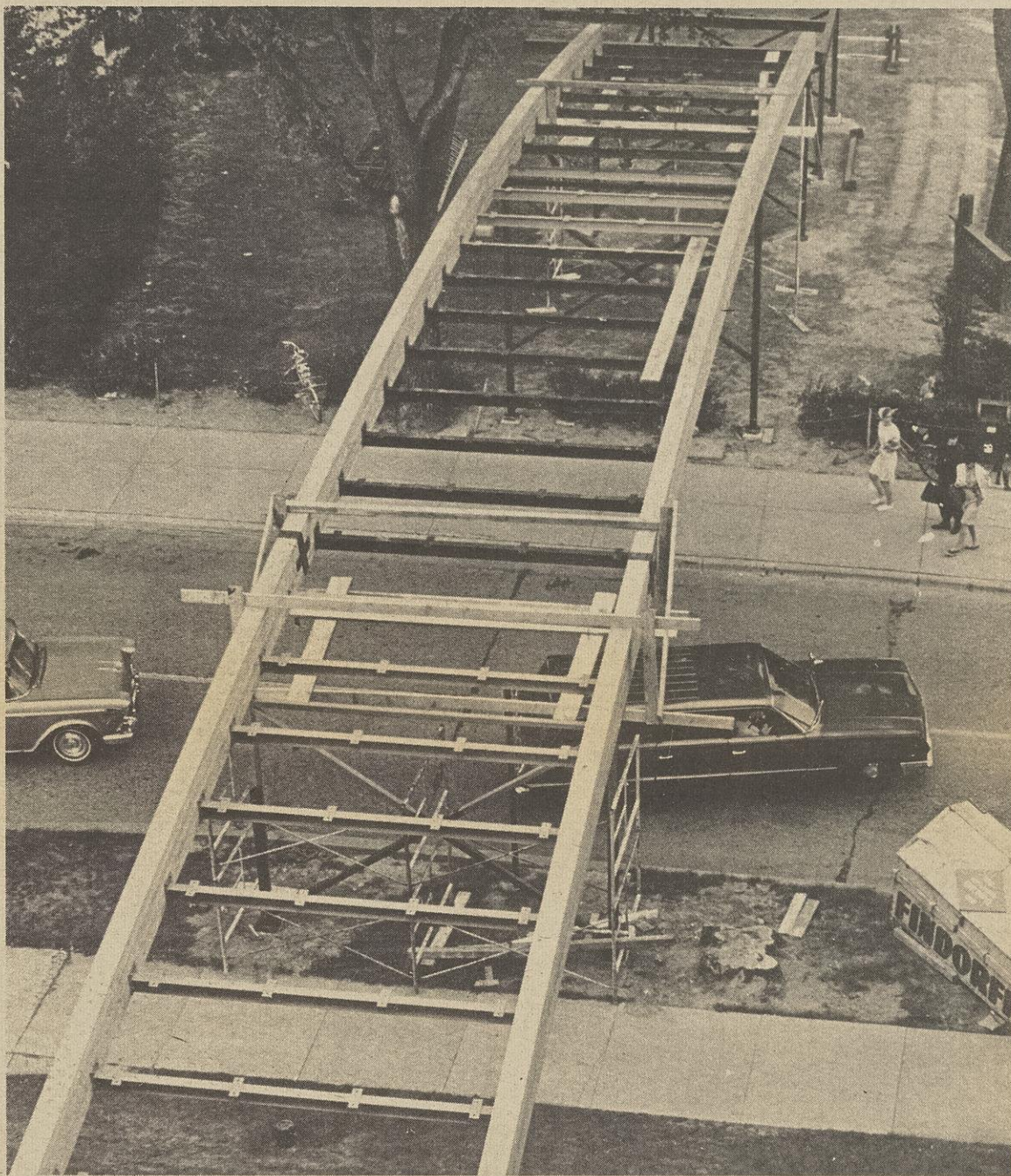
OVERPASS —Two wooden support beams for the second skywalk on the University campus arch across N. Park Street between Science Hall and the Memorial Union just north of the Langdon St. intersection. Heavy pedestrian traffic between classes, often choking off the street to automobiles, made University plans take to the air. The first campus skywalk spans Francis St. between Witte Hall and Gordon Commons.
