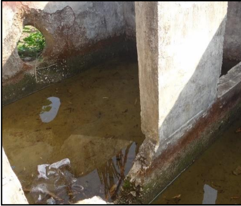
Figure 4.9: Building left from failed government water pipe project. Photograph by P. Vue.
