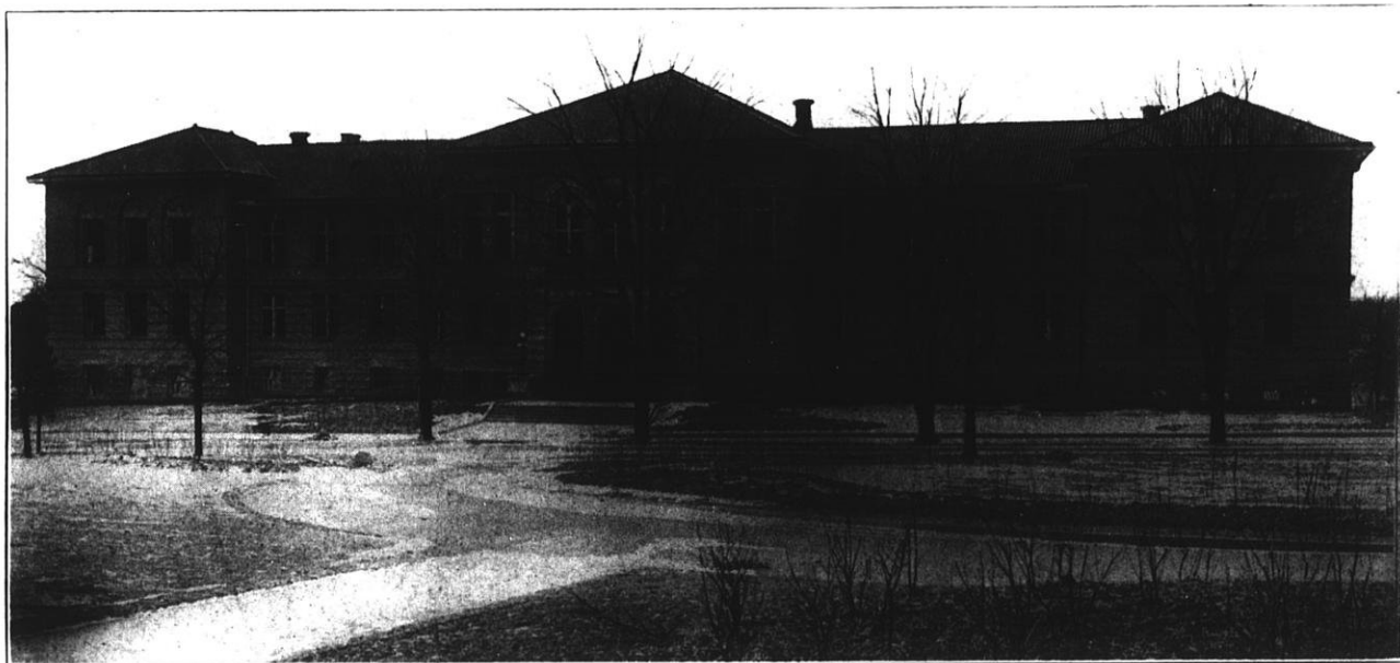
THE HORTICULTURAL BUILDING, OHIO STATE UNIVERSITY
