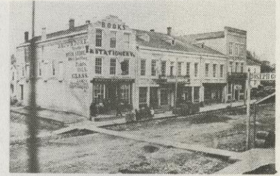
The buildings between Washington Street and Pier Street about 1867 can be seen today by looking at the second story of the buildings now in the block. While the first floors have changed, the upper stories have remained the same.
