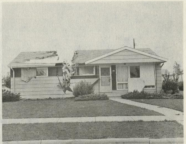
Damage done by the tornado which roared through Port Washington on August 22, 1964, was extensive. This was the Jerry Lorge home at 944 N. Webster St.
