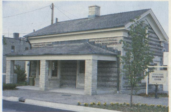
Today the Chamber of Commerce office and information center in the 100 block of East Grand Ave., the Pebble House, a national historic register building, was built in 1848 of pebbles gathered along Lake Michigan's shore. For more than 50 years, where it served as a gatehouse for the power plant. It was moved to the present site in January of 1985 and dedicated on Memorial Day.
