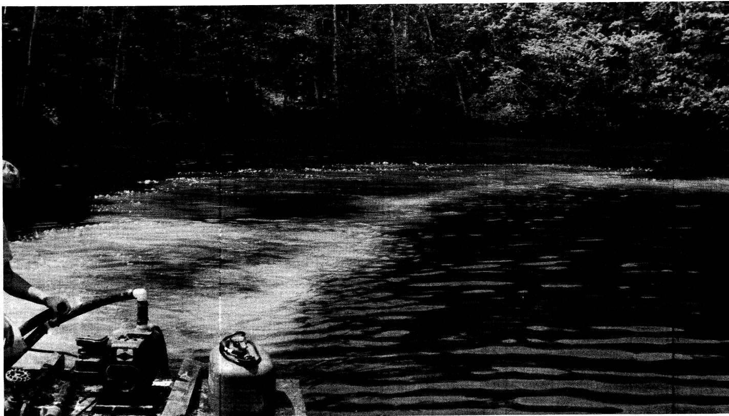
Nutrient inactivation/precipitation at Pickerel Lake, Wisconsin, USA. Liquid alum was applied at the surface and mid-depth by manifold injection. Photo furnished by Peterson (pers. comm.).
