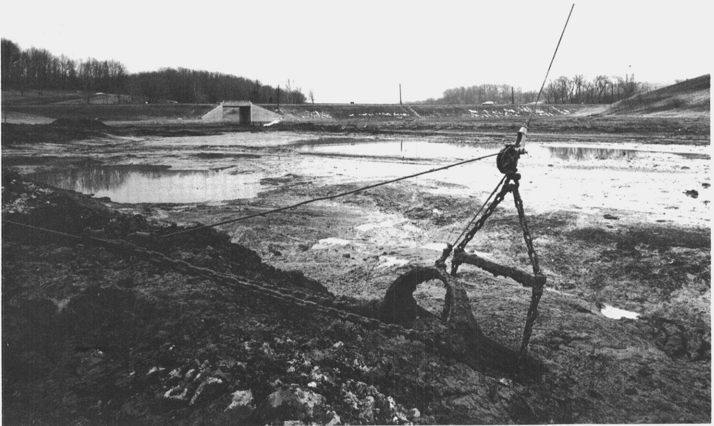
Lake Needwood, Maryland, USA. Flocculant was added to two of the tributaries. After two years of treatment, some 5,600 cubic yards (about 4,300 cubic meters) of flocculated sediment were dredged from this forebay. Photo furnished by McNaught (pers. comm.).
