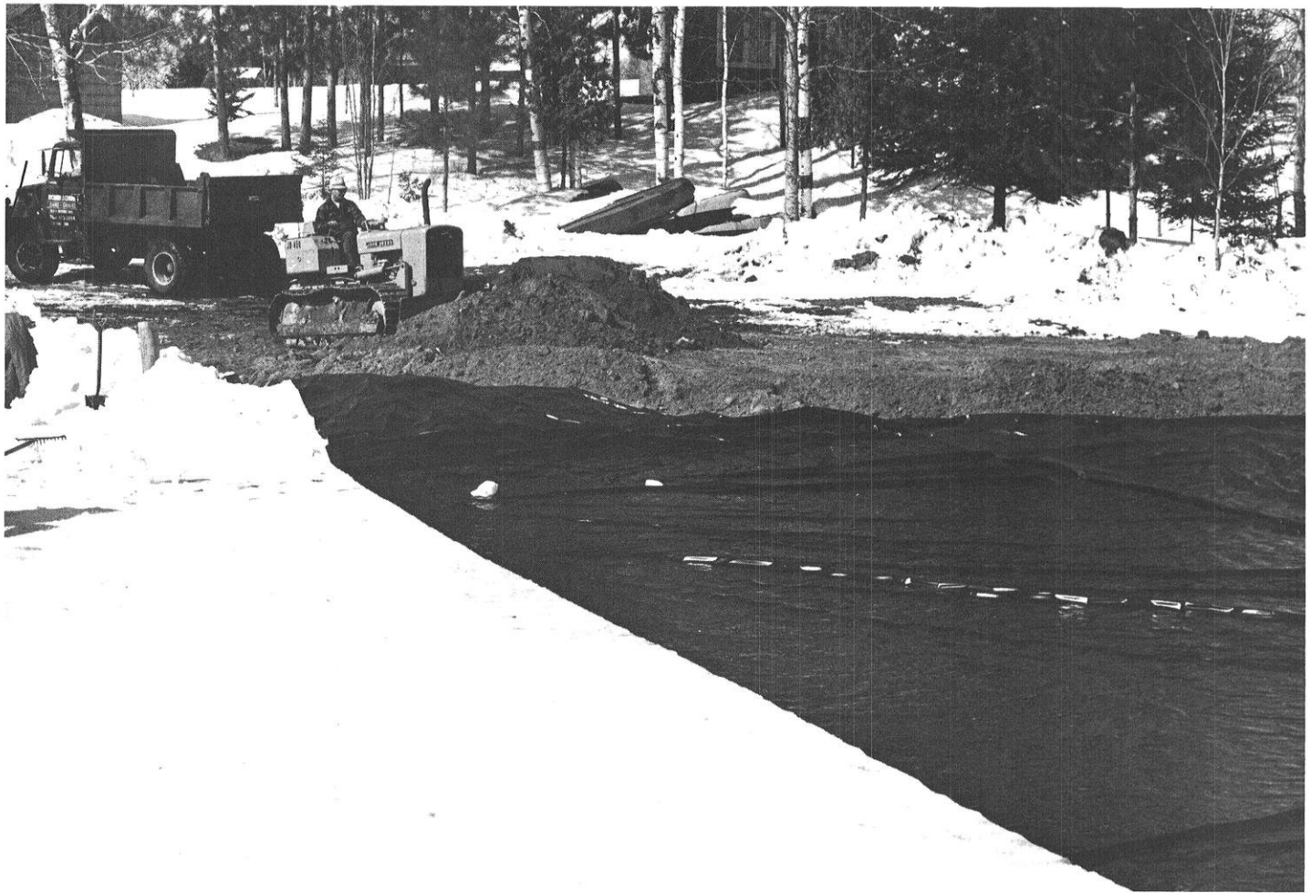
The ice on Windfall Lake, Wisconsin, USA was covered by plastic sheeting overlain with sand. During the spring thaw, the plastic and sand settled onto the lake bottom. Photo furnished by Nichols (pers. comm.).
