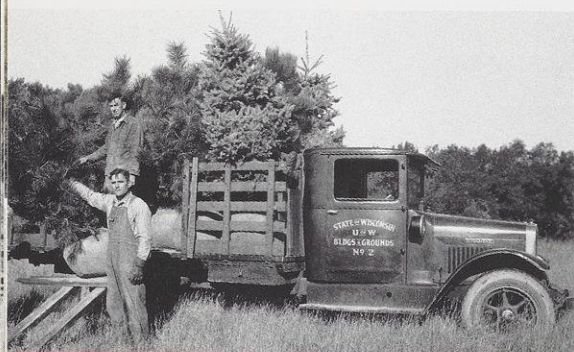
Building the Arboretum, 1934
