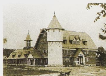
When UW built its dairy barn in 1896 with one of the state's first round silos, we helped make round the shape of things to come.
