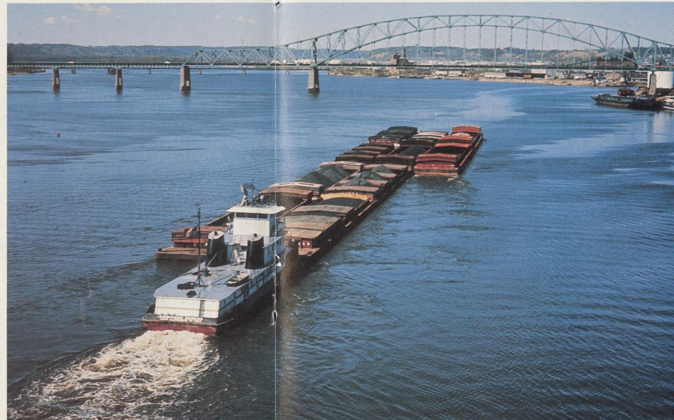
The Wisconsin-Dubuque bridge dead ahead. Towboats and barges move about 67-million tons of cargo per year up and down the Mississippi between Minneapolis and the Missouri River. Wisconsin has river ports at
