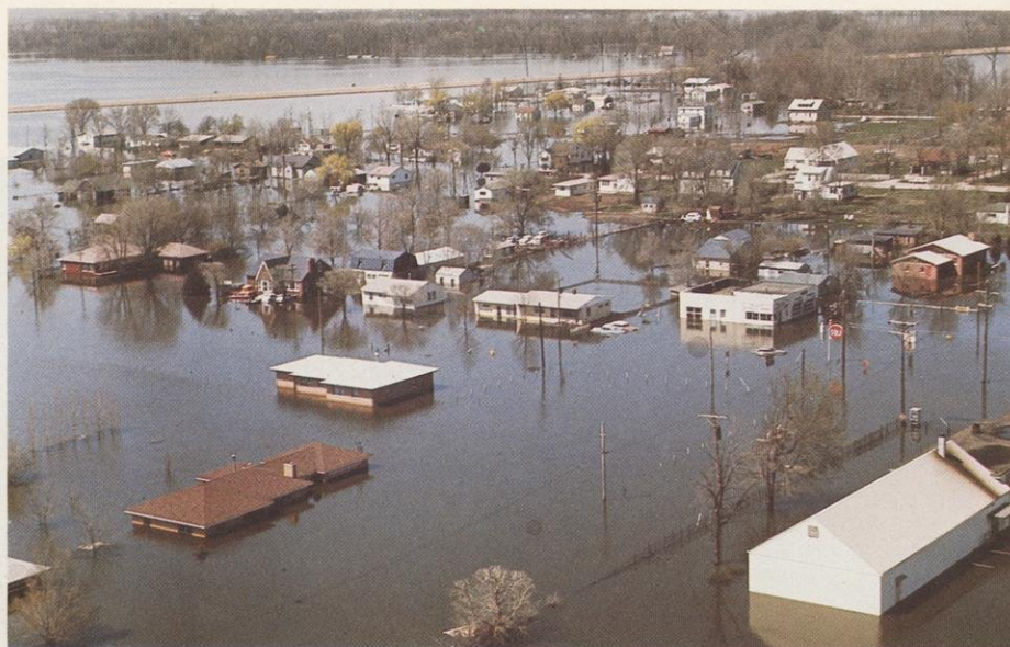
Relocation of buildings to high ground may someday make pictures like this obsolete. Meanwhile, annual damage on flood-prone Wisconsin streams still ranges from about $170 per mile on the St. Croix and Black Rivers to more than $80,000 on portions of the Mississippi, Wisconsin and Trempealeau Rivers. Yearly losses basin-wide are projected to rise from $421-million to $702-million by the year 2000. Major reason is urban encroachment onto floodplains. Photo courtesy of the Minnesota-Wisconsin Boundary Area Commission
