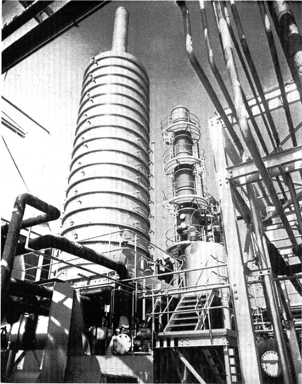
Spires of industry rise above the woods and fields of Kershaw County, South Carolina, where E. I. duPont de Nemours & Company has built the first full-scale commercial plant for manufacturing "Orlon" acrylic fiber in the world. Above are units for recovering essential materials for re-use in the process. See the story on "Orlon and Dacron" on page 17.
