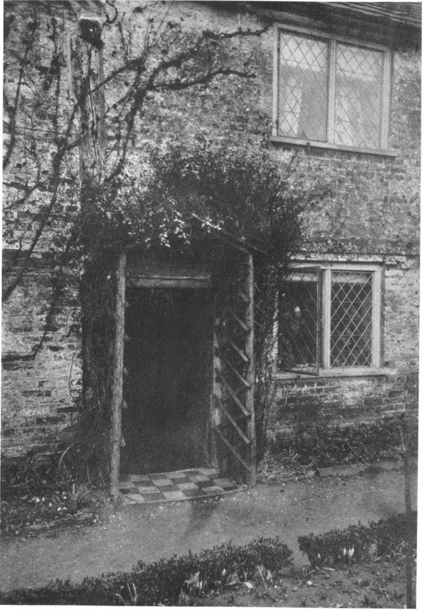
THE DOORWAY OF MILTON'S COTTAGE, CHALFONT ST. GILES, ENGLAND.
