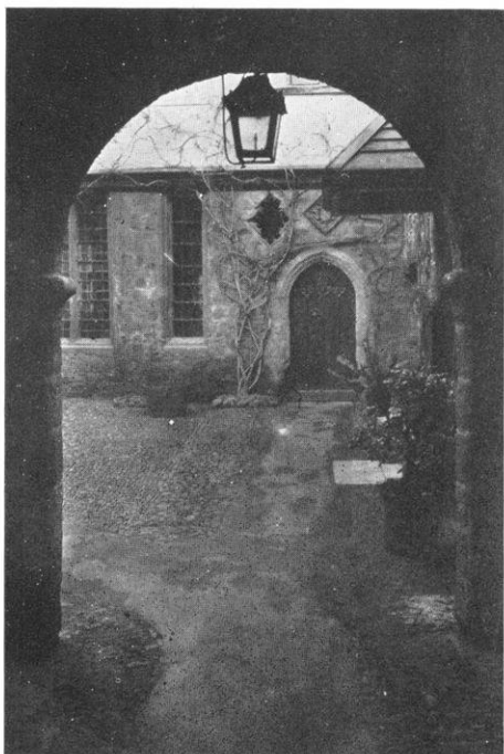
DOORWAY IN THE COURTYARD OF EXETER CATHEDRAL.
